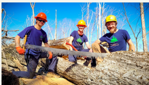
Hurricane spike crew removes hundreds of down trees with crosscut saws in Pond Mountain Wilderness, Tennessee.
