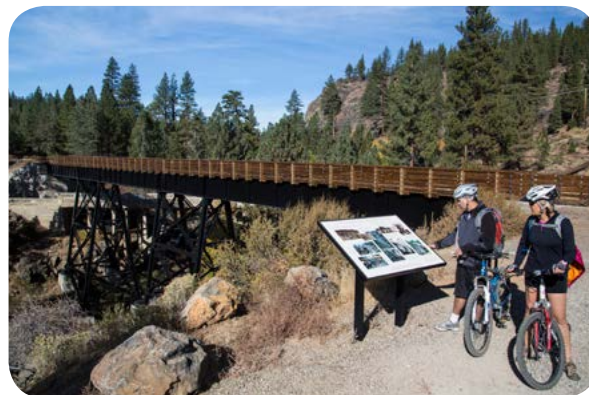
Project converted an old railroad line into a mountain bike trail
